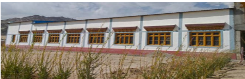
Community Hall developed at Spituk Village of Spituk cluster, Leh
