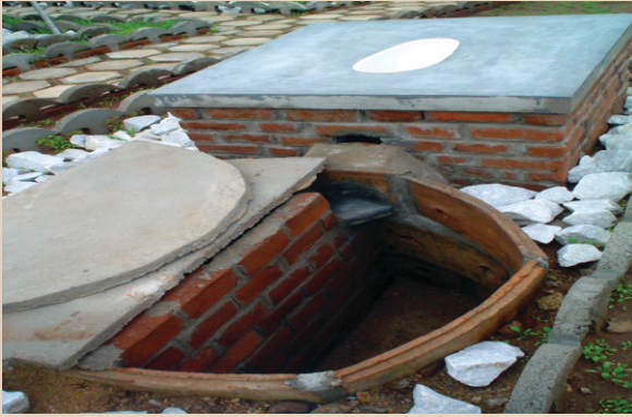
Burnt Clay Segment Leach Pit
