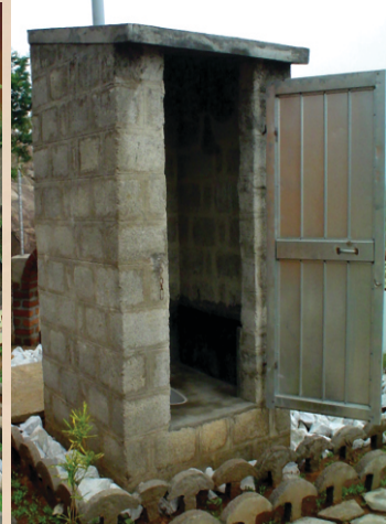
Twin Pit Latrine with Pre cast Concrete Blocks
