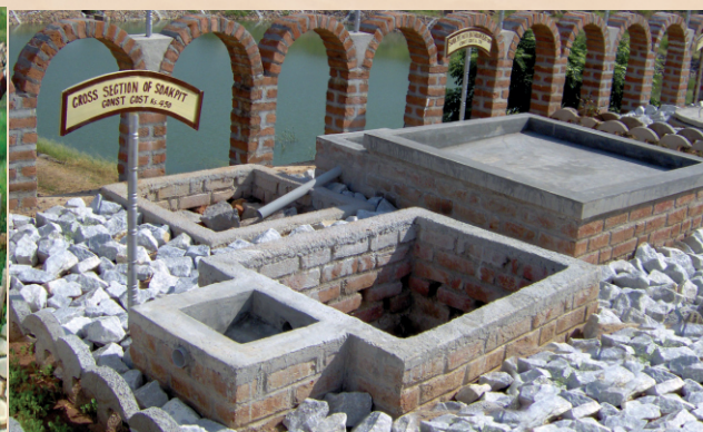
Soak Pit for Bathroom Platforms
