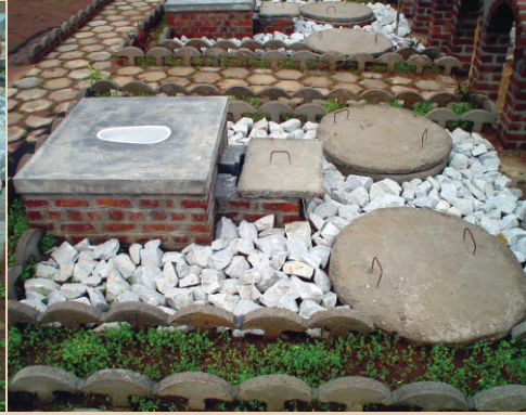
Circular Twin Pit Toilet with Bricks
