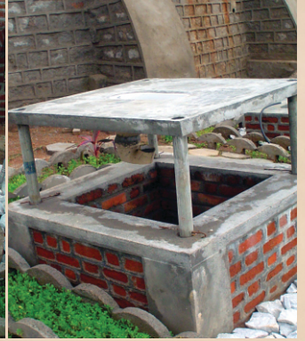
Single Leach Pit Toilet with P-trap Pan
