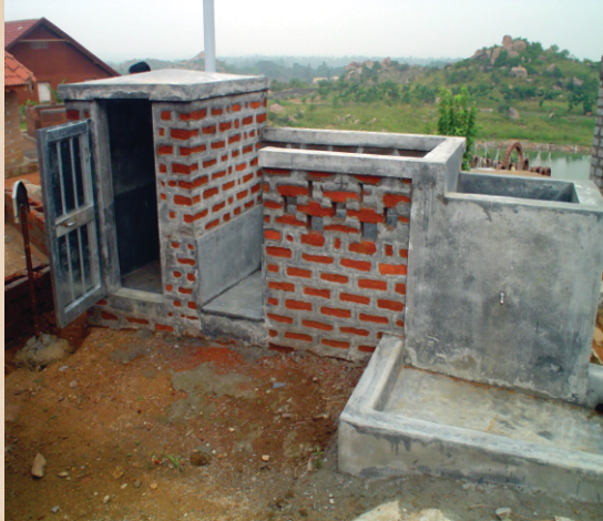
Anganwadi Toilet Block
