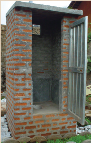
Two Pit Latrine with Flap Seal Pan and Brick Work
