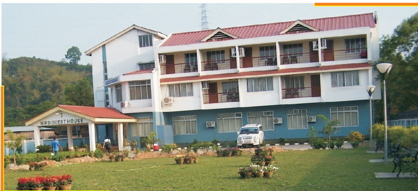
A view of new hostel (Brahmaputra)
