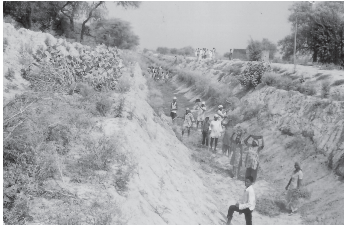
Desilting work of Minor Irrigation Canal in Progress in district Sirsa
