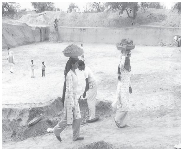
Pond Excavation work in progress in district Mahendergarh
