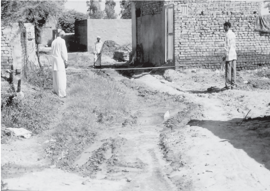
Gali Construction in Harijan Basti under NREGS
