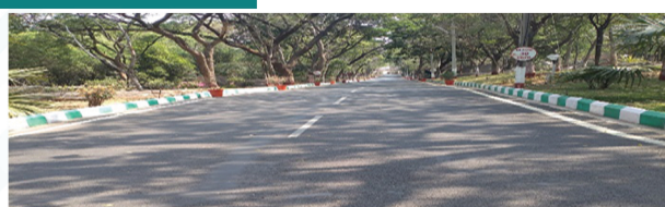
NIRDPR Campus Road laid using waste plastic
