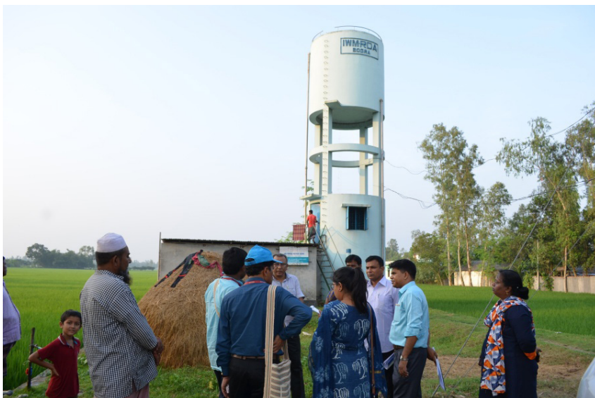
Integrated Water Management Project, RDA, Bogura
