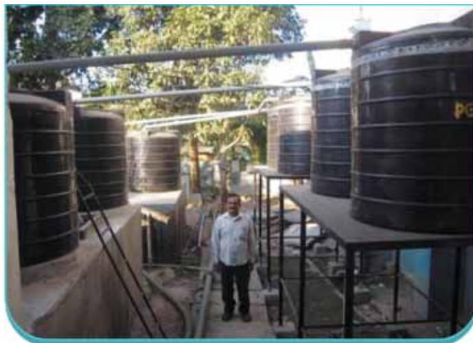
Water storage tanks (left) and filtration tanks (right)
