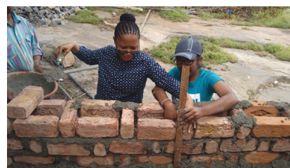
Construction of rat-trap walling
