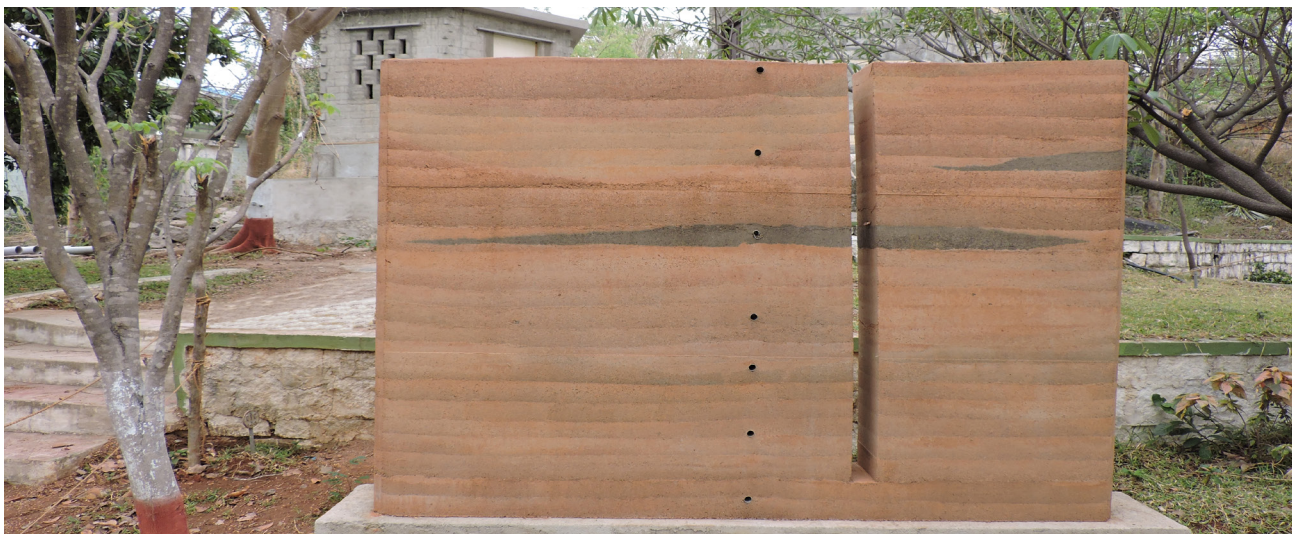
A demo wall constructed using rammed earth technique at Rural Technology Park, NIRDPR
