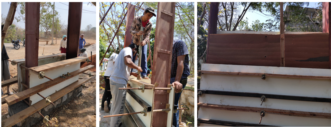
Various stages of rammed earth wall making
