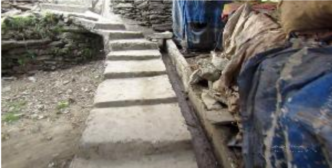
Concrete drain alongside village path
