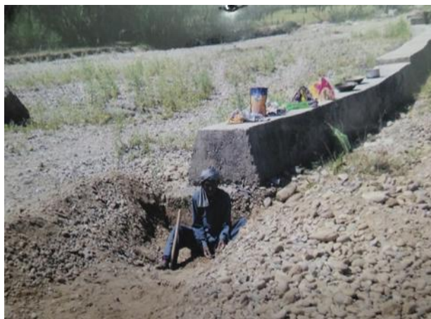
Construction of spar and retaining walls to protect agricultural land from soil erosion during floods
