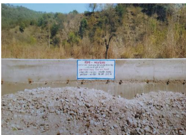
Construction of spar and retaining walls to protect agricultural land from soil erosion during floods
