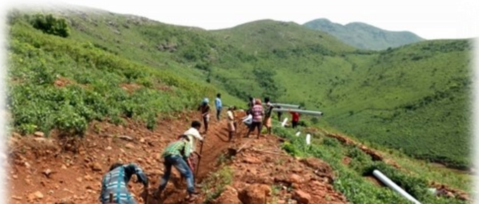
Work on spring-based irrigation in progress at Putsil village, Koraput district, Odisha
